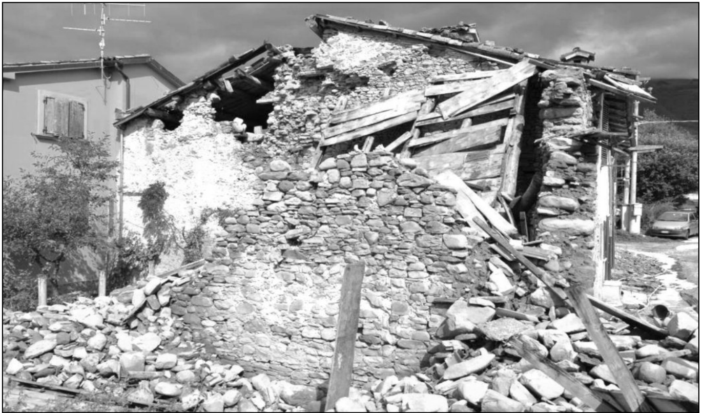
Figure 1 - Masonry building made of irregular shaped stones, with poor quality ground soil mortar, partially collapsed (neighbouring of Amatrice, photo credits: Author 2016)
