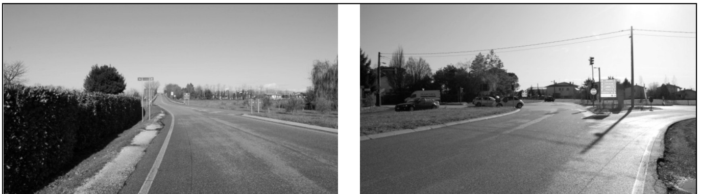
Figure 4 - Segment 1D: intersection with the SS 14 motorway looking north (Fogliano Redipuglia) and south (San Canzian d’Isonzo)
