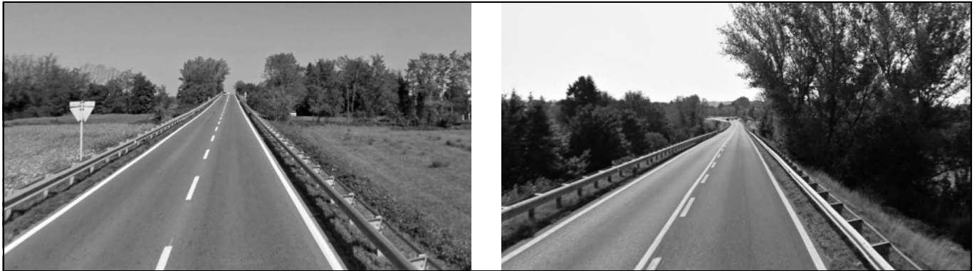
Figure 5 - Segment 1D: the initial segment looking north (Fogliano Redipuglia) and south (San Canzian d'Isonzo)
