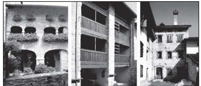
Figures 4, 5 - The “ ballattoio su setti ” type typical of Andreis in an isolated building and within a row (Chinellato et al., 2002).
