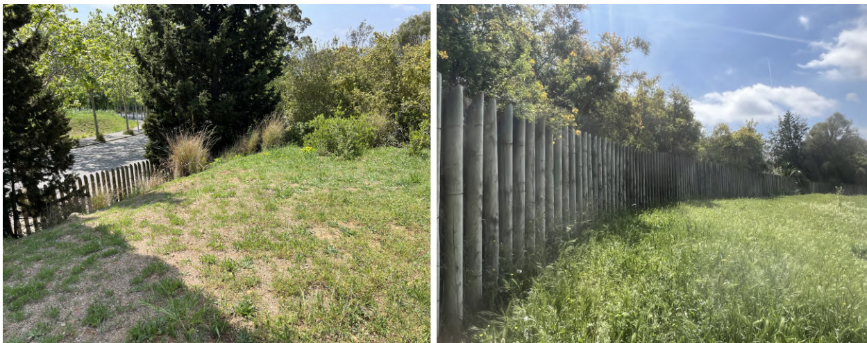
Figure 9. Enclosure along the edges of the Barcelona Botanical Garden. Photo by author.
