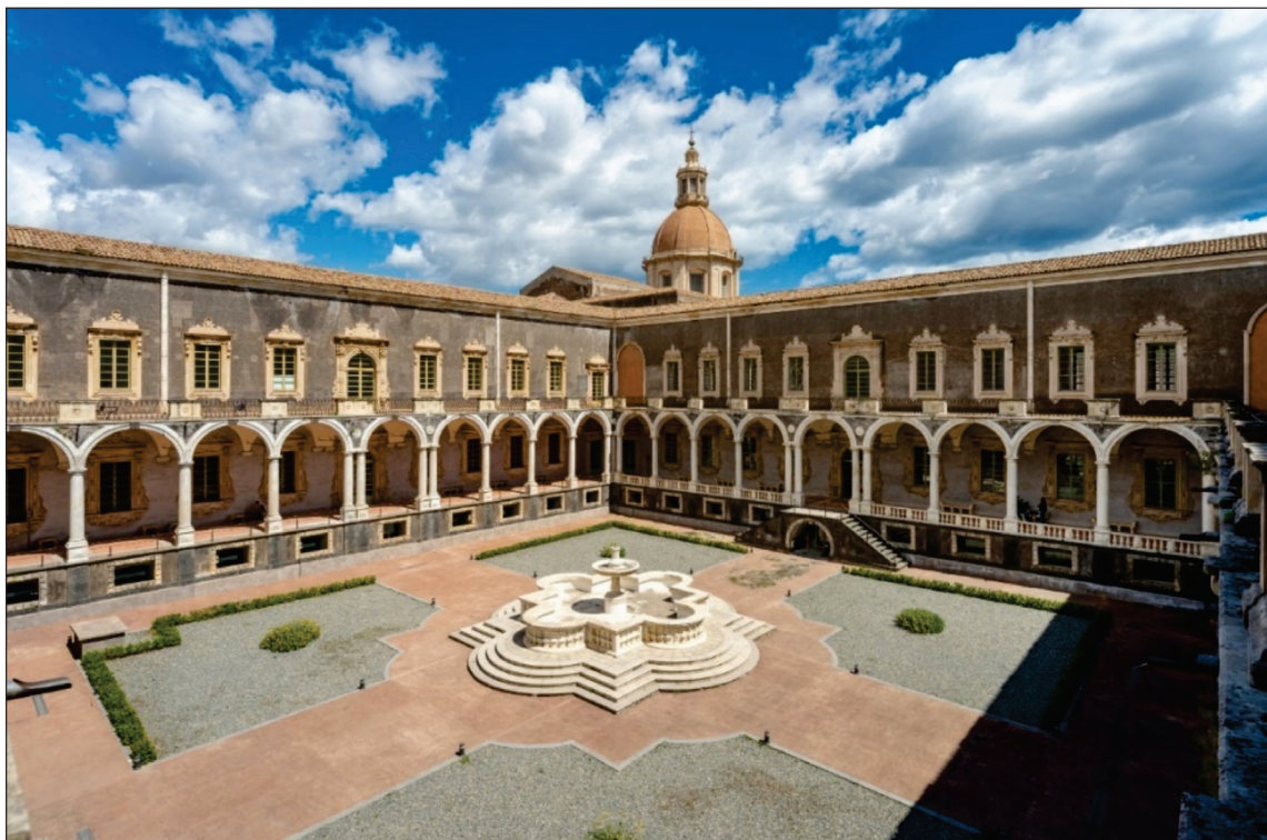
Figure 1. Photograph of the Northern Cloister of the Benedictine Monastery in Catania
