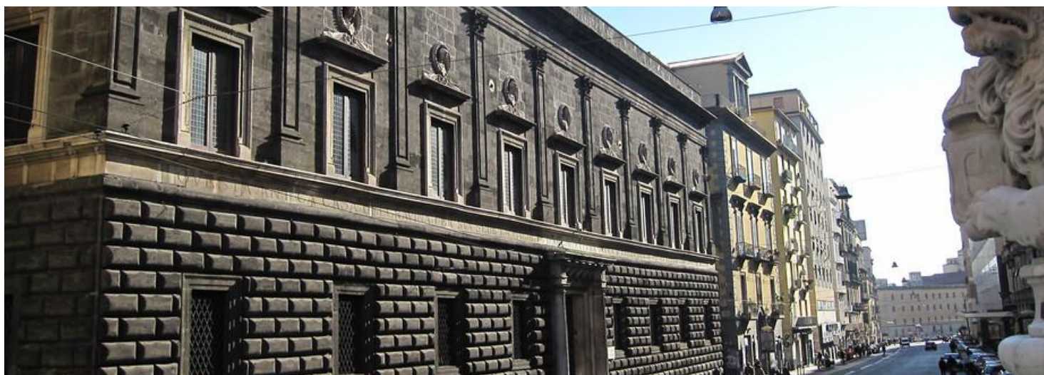
Palazzo Gravina (Via Monteoliveto 3 – 80134, Naples, Italy).
